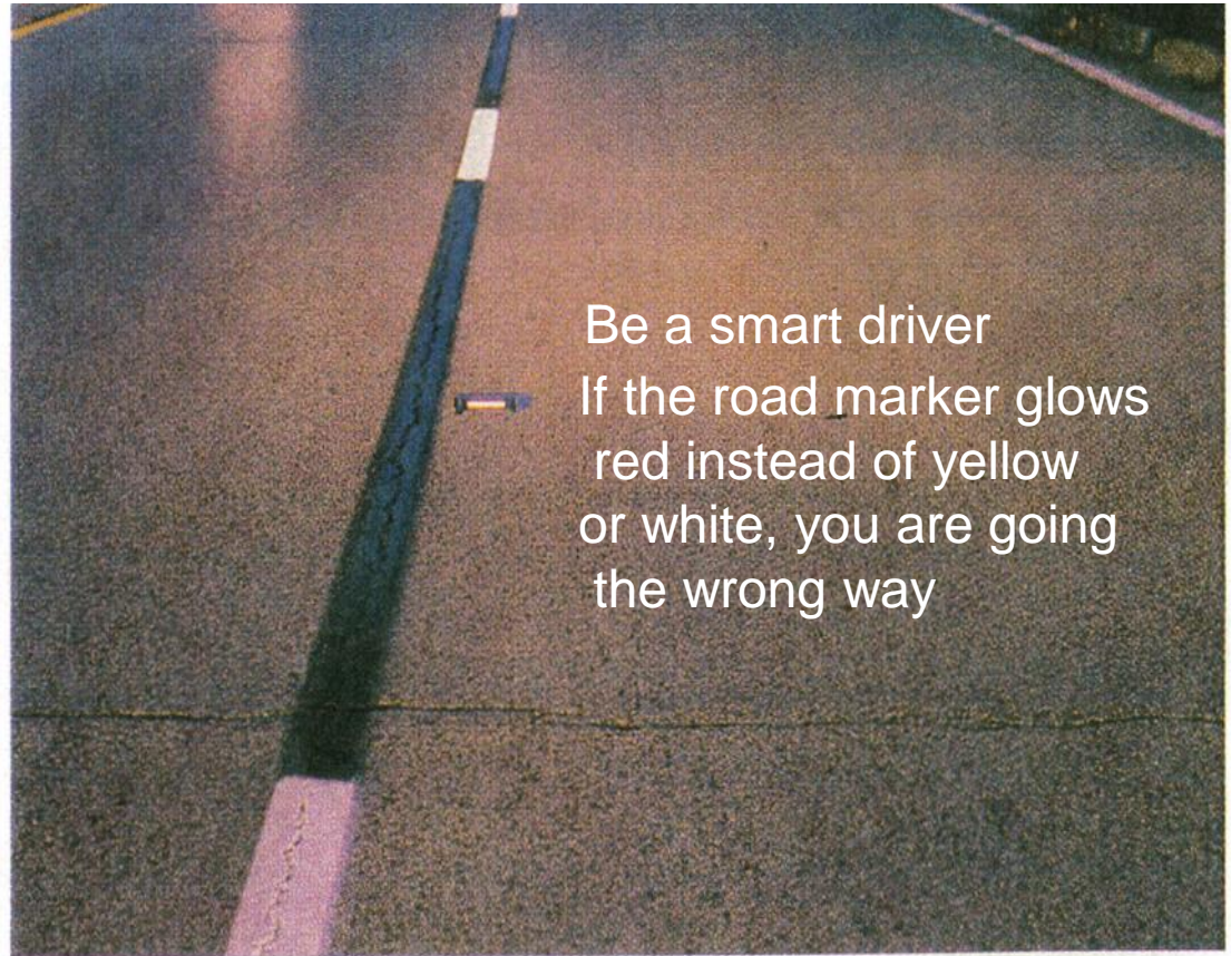
Roadway markers shine when struck by headlight beams to help drivers see the driving lane at night.
